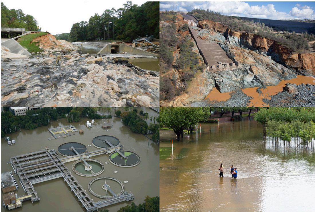
Fig. 1. Recent flooding has decimated infrastructure and left thousands homeless. In October 2015, Hurricane Joaquin caused widespread flooding in South Carolina and destroyed Cary Lake dam in Columbia ( Upper Left ). Heavy rain and flooding caused the Oroville Dam spillway in northern California to fail in February 2017 ( Upper Right ). And in August 2017, massive rains from Hurricane Harvey spurred extensive flooding across much of Houston ( Bottom Left and Right ). Images courtesy of Hermann Fritz (Georgia Institute of Technology, Atlanta) ( Upper Left ), The California Department of Water Resources ( Upper Right ), Shutterstock/DIIMSA Researcher ( Lower Left ), and Shutterstock/michelmond ( Lower Right ).
